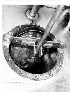
ROD OF HANDLING TOOL, resting on a metal fixture, supports 68-pound boiler cover after it has been removed from its position inside the boiler.
